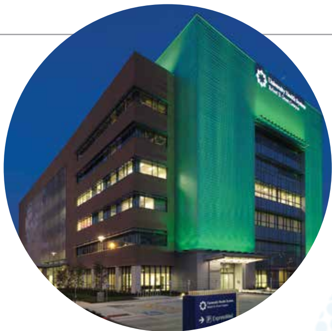
The technologically advanced new building on the Robert B. Green Campus downtown opened in early 2013.
