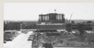
Construction gets underway for the South Texas Medical School.
