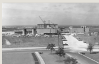
Ground is broken for the $15 million Bexar County Hospital.
